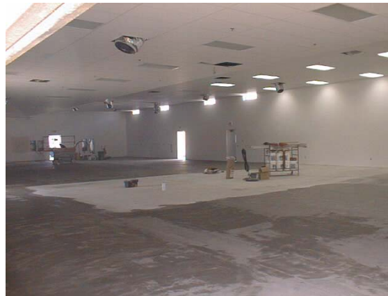
7200 ft² experimental space is being refurbished for use in IFE research
